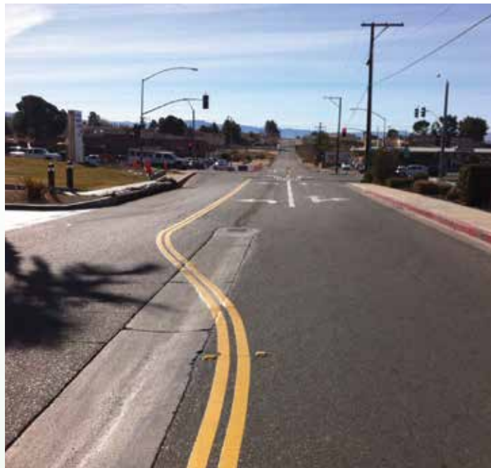
Looking south on Kasota Road at Highway 18, separating the left turn and through lanes has greatly improved traffic in the area
