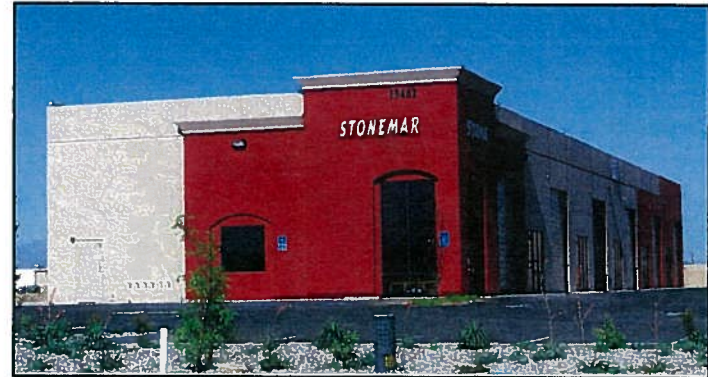
This commercial development stands along Central Rd.
