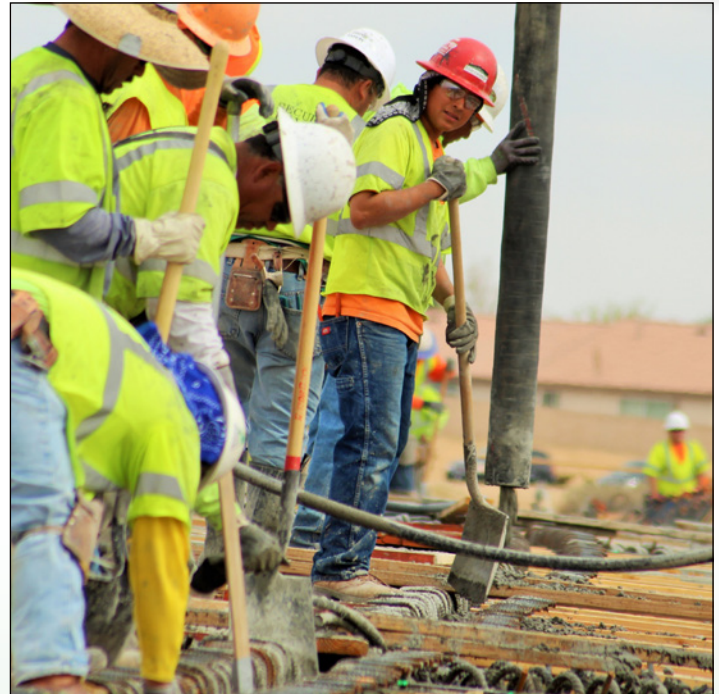
The first concrete was poured at the Yucca Loma Bridge on March 16. In 12 hours, three teams directed 213 trucks and poured 2,130 cubic yards of concrete. Visit www.YuccaLomaBridge.com to view live images from the construction site, 24 hours a day.
