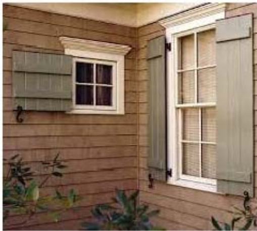
Shutters (faux shutters)
