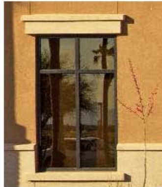
Lintel over Window
