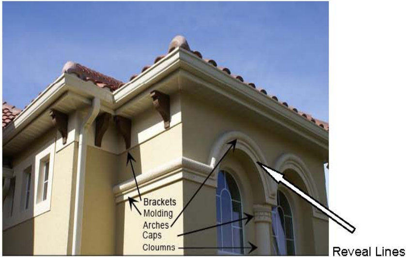
Molding with "Reveal Lines"
