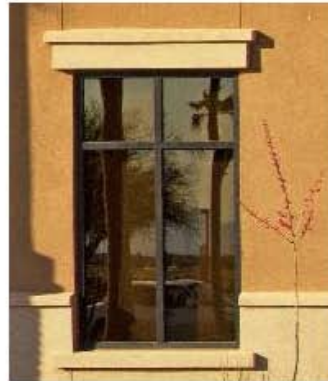
Lintel over Window
