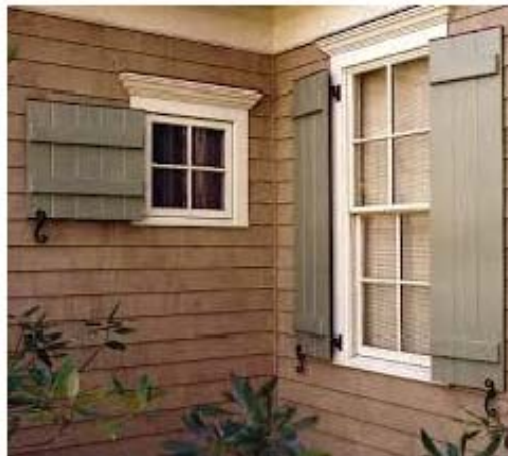
Shutters (faux shutters)
