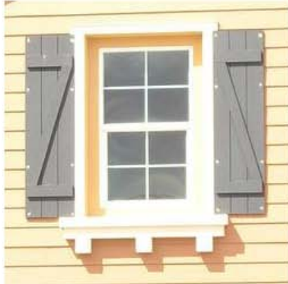
Corbels under Window Sills (decorative)
