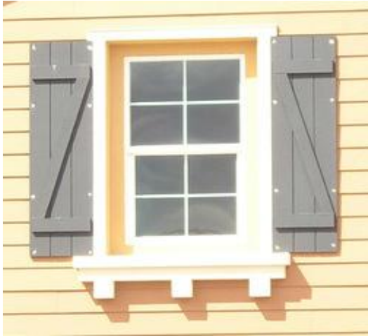
Corbels under Window Sills (decorative)
