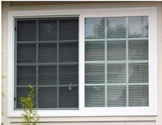
Windows with Mullions Sash Transom, Muttons and Architrave
