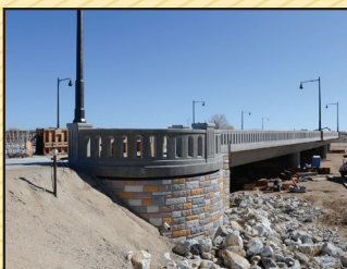
Yucca Loma Bridge NEARLY COMPLETE...Pg. 12
