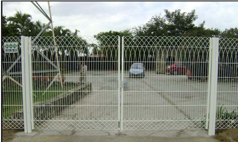
This is the fence type presented by the Council Member. It is powder coated wire and comes in panel sections. The design includes asymmetrical interlinked loops.
