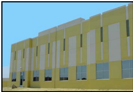
Typical Tall Building
