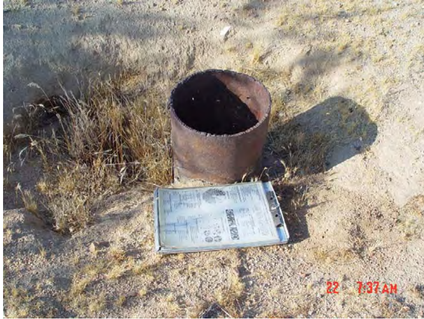
11. Abandoned well casing in southwest corner of Site.
