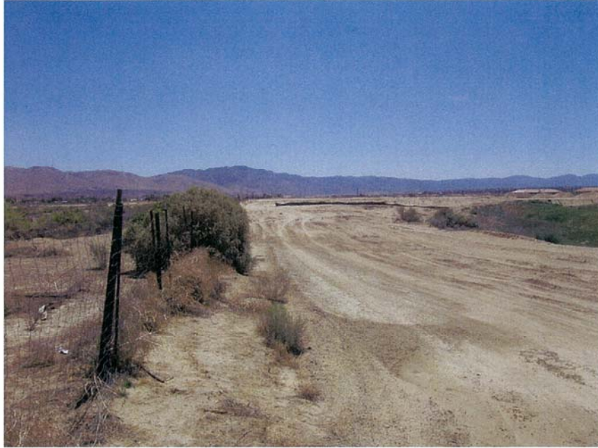
NWC – LOOKING SOUTH AT CONSTRUCTION SITE (September 2004)
