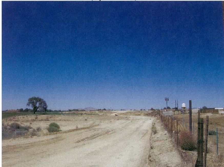
NWC – LOOKING NORTH ALONG GOLF COURSE AND CONSTRUCTION SITE (September 2004)
