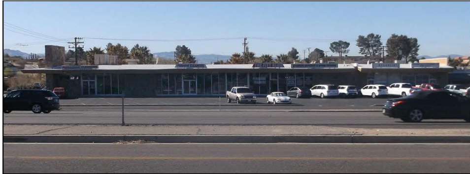
Figure 7. Commercial buildings at 18155-18157 and 18165-18195 Outer Highway 18 South, view to the south. (Photograph taken on March 13, 2018)
