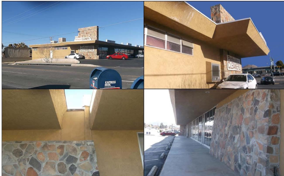
Figure 8. Primary and eastern façades of the 1955 building at 18165-18195 Outer Highway 18 South. Clockwise from top left : fieldstone “tower” at the northeast corner of the building, view to the southwest; extended, angled eave over drive-up banking window, view to the northwest; fieldstone panel and plate glass windows in the front façade, view to the east; close-up of the junction between the two buildings. (Photographs taken on March 13, 2018)
