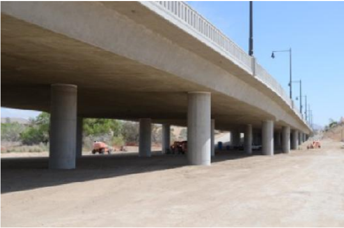
The long awaited Yucca Loma Bridge nearing completion.
