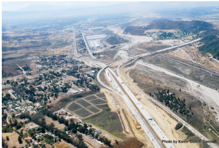
I15-215 Devore Interchange Project
