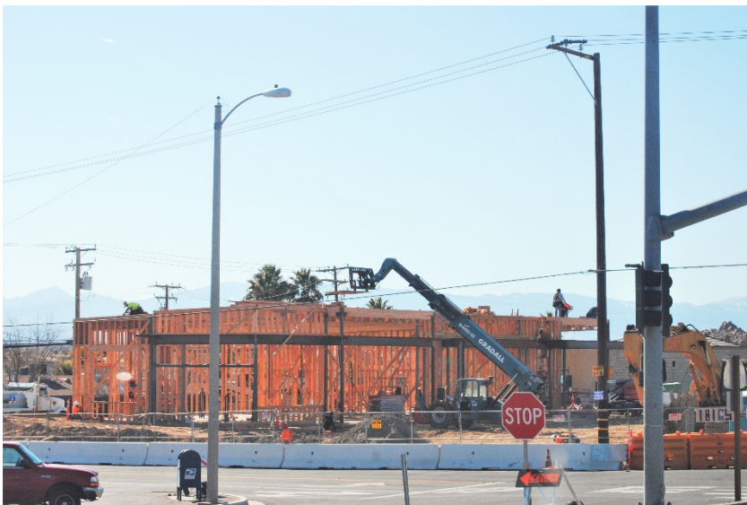
New Starbucks under construction
