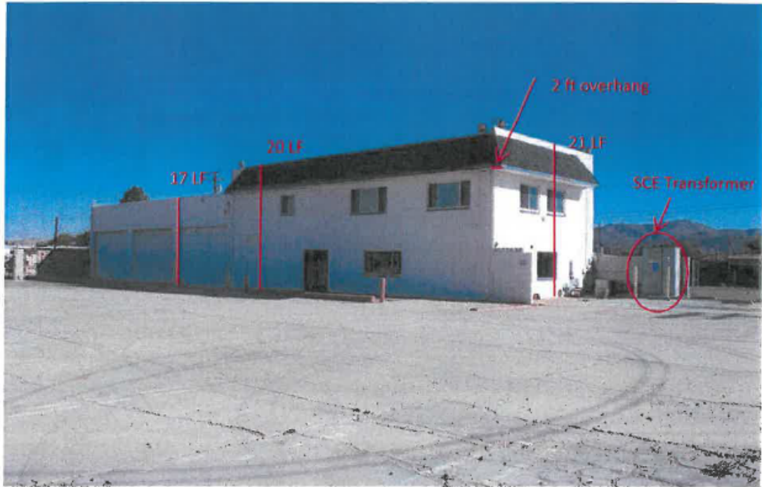
Exterior building view looking north-east
