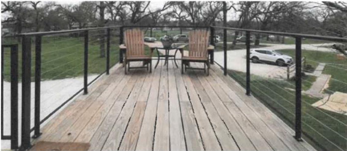
Steel railing post and stainless steel cable guardrails. Post and top rails to be Grey.
