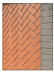
STAMPED COLORED ASPHALT PAVING
