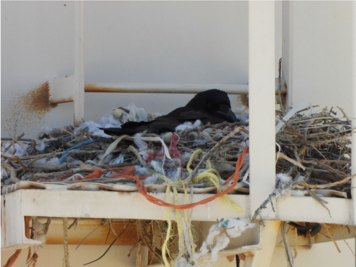
Photo 1: Common Raven nest on water tower southeast of the project site.
