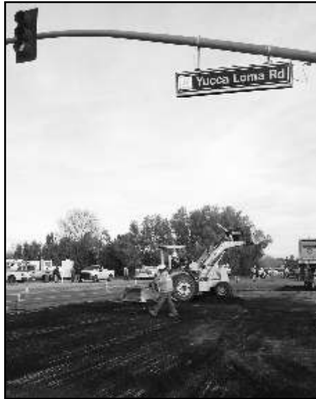
Work began January 3 on repaving from Yucca Loma to Highway 18.
