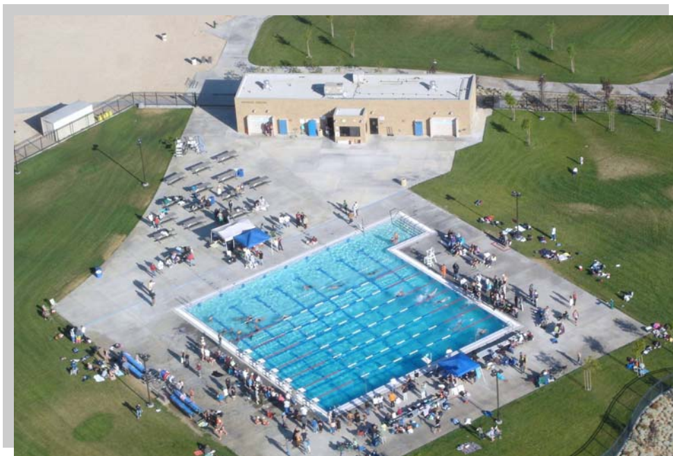
Civic Center Park Aquatic Center
