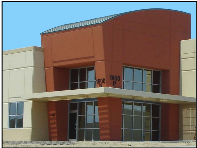
Typical Building Entry
