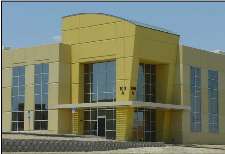
Typical Windows and Doors
