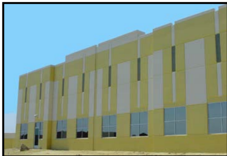
Typical Tall Building
