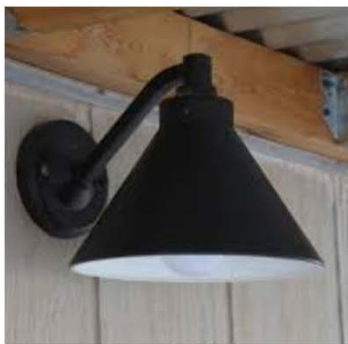
Examples of shielded lighting
